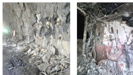
① Failure of side arch ② Failure of bus tunnel entrance
