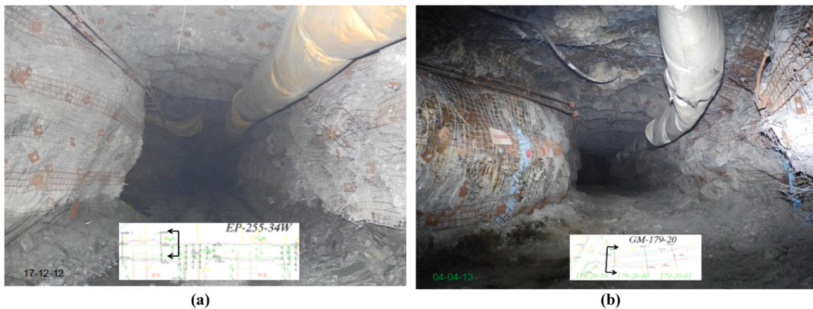
Fig. 32. Squeezing conditions in La Ronde and Lapa mines in Canada: (a) pronounced squeezing, 2550 m depth; and (b) pronounced squeezing, 1790 m depth [297].
