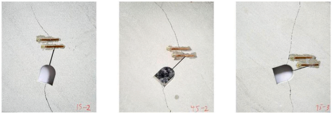
Fig. 24. The crack patterns from tests.
