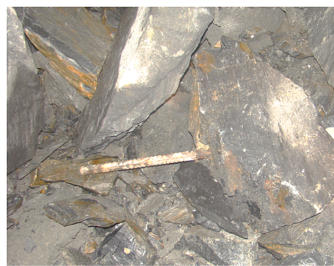
Fig. 13. The local surrounding rock occurred shear deformation of the middle wall between Jinping II underground powerhouse [7].
