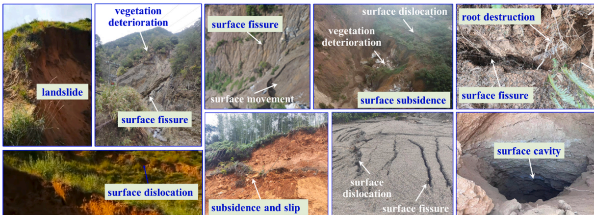
Fig. 6. Common surface damage caused by mining.
