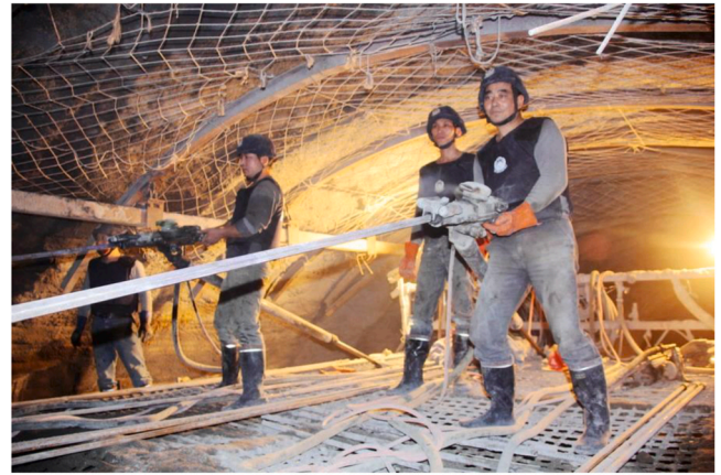
Fig. 22. Workers are equipped with bullet-proof vests and helmets to work in the strainburst-prone Micangshan Tunnel of the Bashan-Shaanxi Expressway (photo source: www.guancha.cn ).
